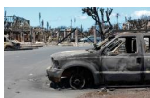
Damaged buildings and vehicles in Lahaina. [Sp. Sean Walker, photo.]
